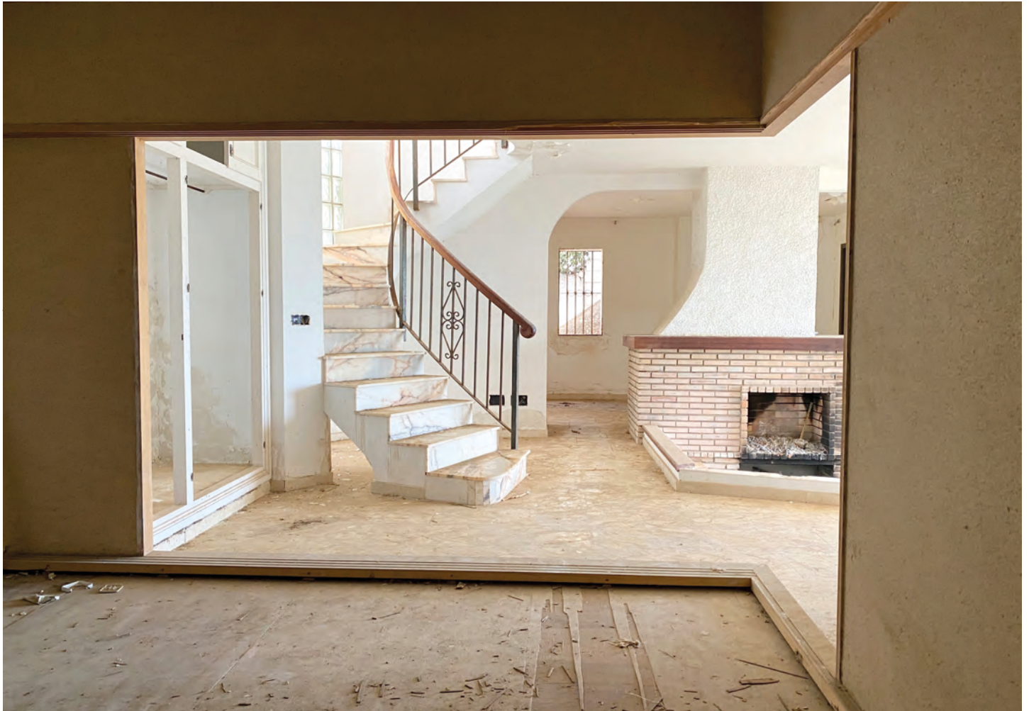
Figure 11. Third house built in 1987. Japanese style room interior, connected to the western style living room with chimney and built-in bench. The floor used to be tatami type, but as can be seen in the picture taken by the authors in October 2021, it is in need of urgent repair.
