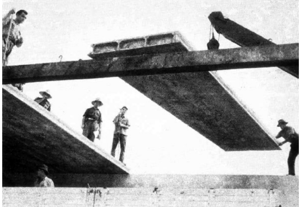
Figure 1. Horpresa panel from the Bahia Bella house prototype. Image from Hogar y Arquitectura , n. 64, 1966. © Fundación Alejandro de la Sota.
