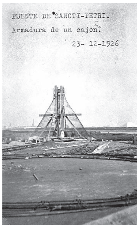
[Fig. 11] “Sancti-Petri bridge. Support reinforcement 23.12.1926”. Source: Torroja archive, CEHOPU-CEDEX, I-ETM-018-01_01.
